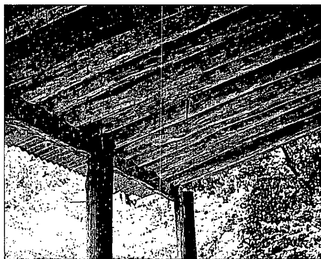
These verandah roof timbers are the curved 'flitches' from 2.4-metre railway sleeper logs that Stu Anderson bought "almost for nothing" from a local mill.
